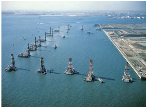
Sea-bed Improvement Works by Specialized Vessels for Sand Compaction Pile Method
