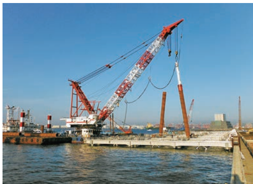
Steel Pile Driving Works
