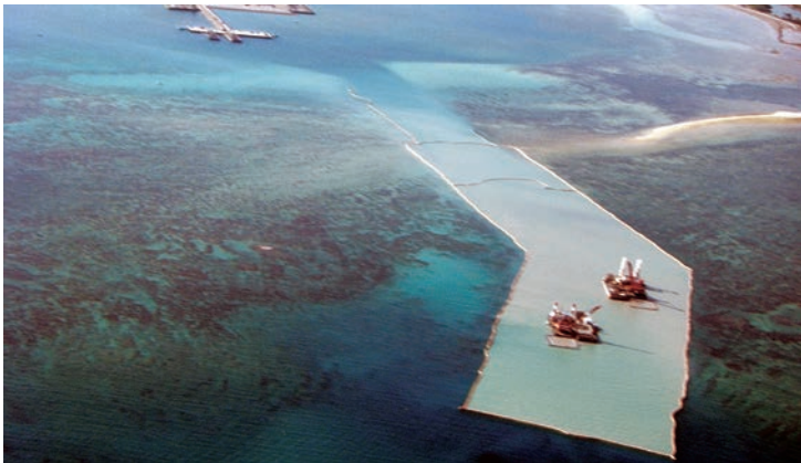
Dredging Work with Sheet Protectors for Protecting Sea Pollution by Dredged Soil (Okinawa Nakagusuku Port)
