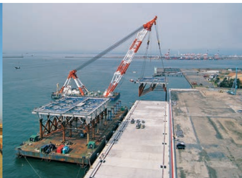
Installation Work of Steel Jacket Structure
