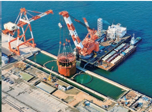
Installation Work of Steel Sheet Cellular Structure
